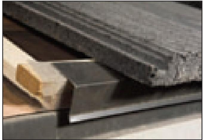
*Alternative eave installation utilizing a counterbatten system or risers, provides under tile ventilation. A ridge vent can be installed as well in order to exhaust air pulled in through the eave. Solar Panels perform optimally when well ventilated and cool.*
