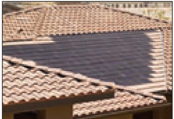
*Alternately, Bel Air can be mixed with Capistrano. Capistrano can make up the majority of the field tile, while Bel Air may be installed around the solar roofing tiles.*
