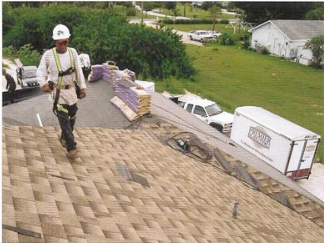
Kelly Roofing deals exclusively in larger-exposure shingles such as Elk's Prestique Grandé.
